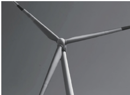
wind blade deformation inspection
